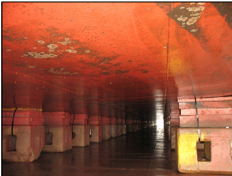
Figure V. 2: Vessel on dry dock blocks. The rectangular blocks suspend the vessel for maintenance, repair, and paint re-application.
