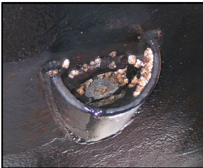
Figure V.1: Intake opening on a vessel hull.
